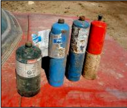
Prohibited: Propane, butane & acetylene bottles
