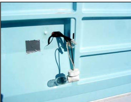
Removing mercury switch in a freezer
