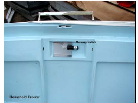
Mercury switch in a freezer
